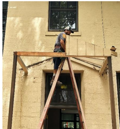
Old entrance to the novitiate being dismantled; a new design will go up
